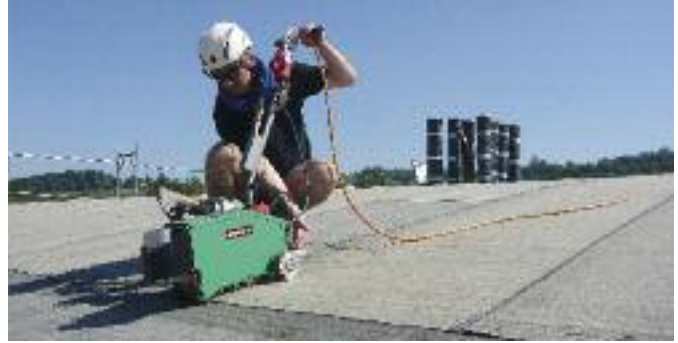
Flameless modified bitumen welding with the BITUMAT B2.
