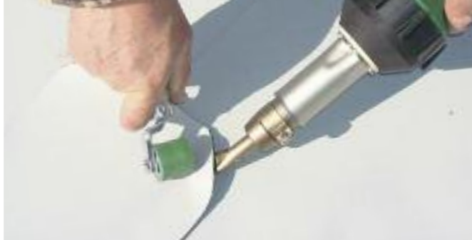
TRIAC S while overlap welding on the roof..
