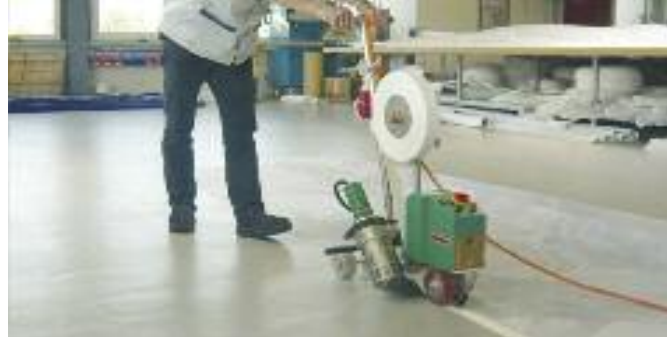
Welding tape at maximum speed.
