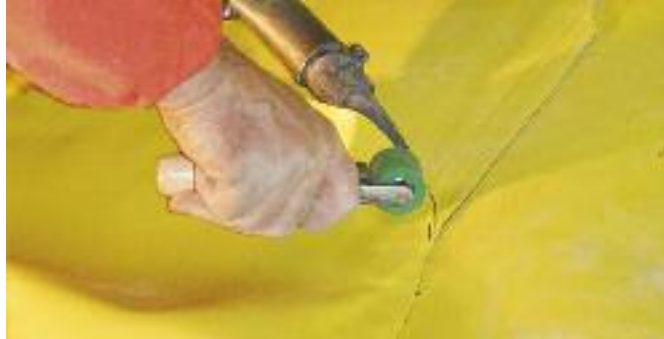
The hand pressure roller is an essential accessory for tunnel applications.
