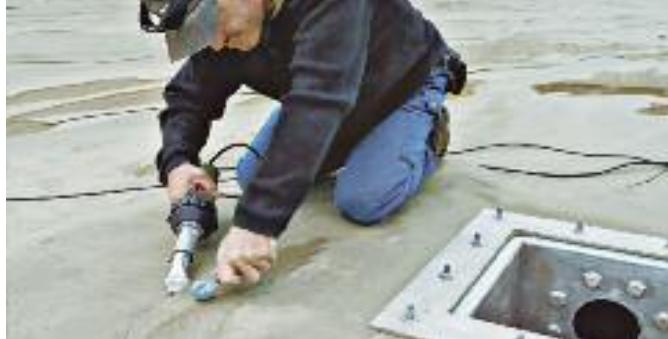
TRIAC S in use welding a future a storage reservoir.
