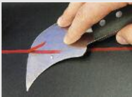
Step 4: Planing the projecting welding rod with the spatula. (page 34)
