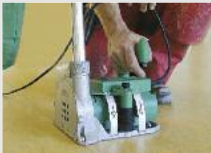
Step 1: Milling the groove with the GROOVER. (page 91)
