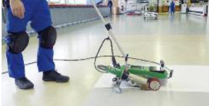
Constant, wrinkle-free overlap welds.
