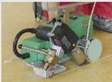
Step 2: Inserting the welding rod into the groove with the UNIROOF E hot air welder. (page 90)
